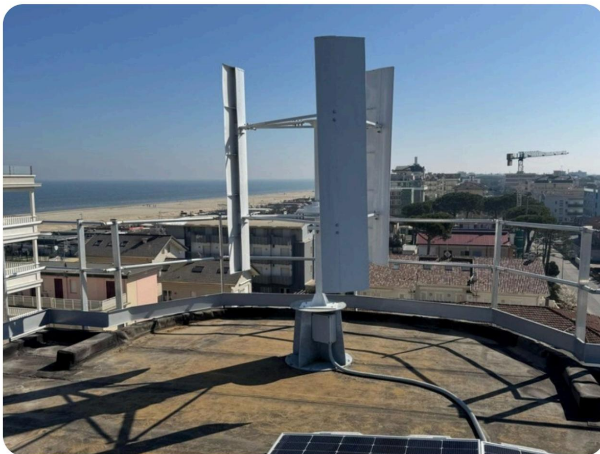
INSTALLATION OF 4 3KW TURBINES COMBINED WITH A SYSTEM 60KW PHOTOVOLTIC SYSTEM AT THE VILLA DEL MARE HOTEL IN CERVIA
