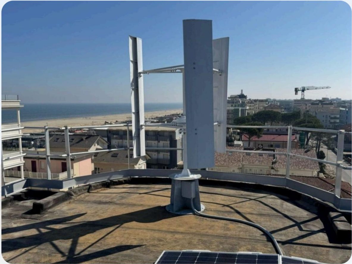
INSTALLATION OF 4 3KW TURBINES COMBINED WITH A SYSTEM 60KW PHOTOVOLTIC SYSTEM AT THE VILLA DEL MARE HOTEL IN CERVIA
